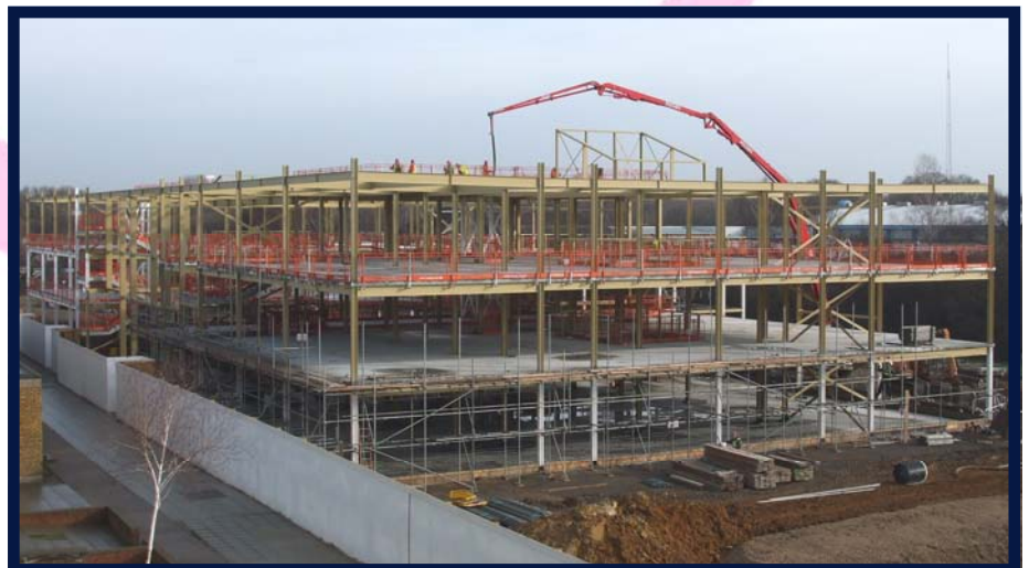
Pictured above: Current progress of building work at Oasis Academy Mayfield
